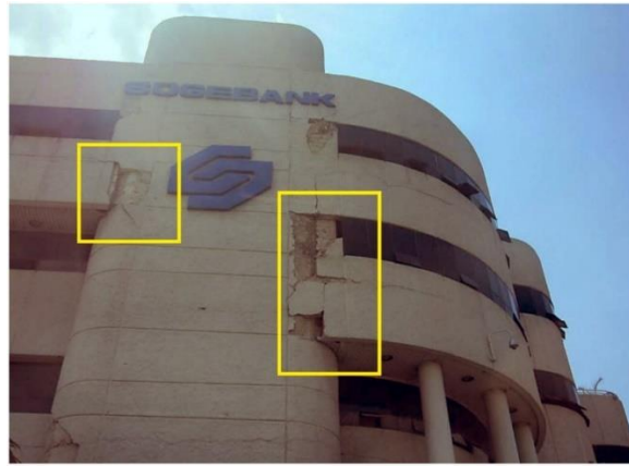
Figure 5 Cracks detected by the approach suggested by Young-Jin Cha and Wooram Choi
