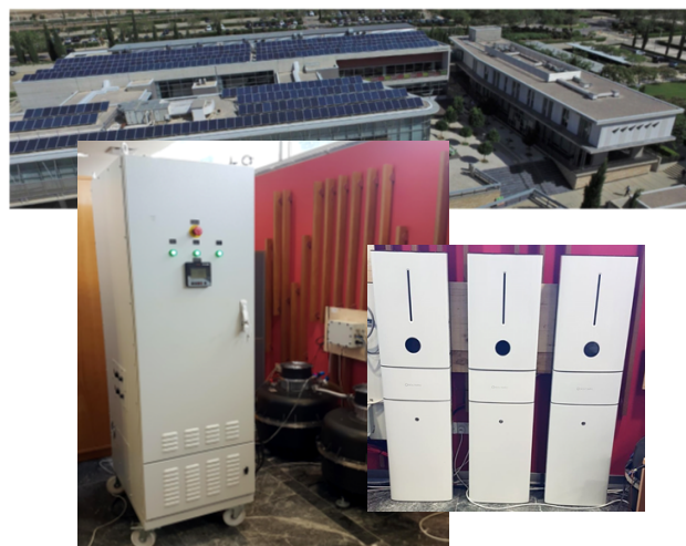
Pilot II: Battery & Flywheel storage system at KIOS CoE (UCY)
