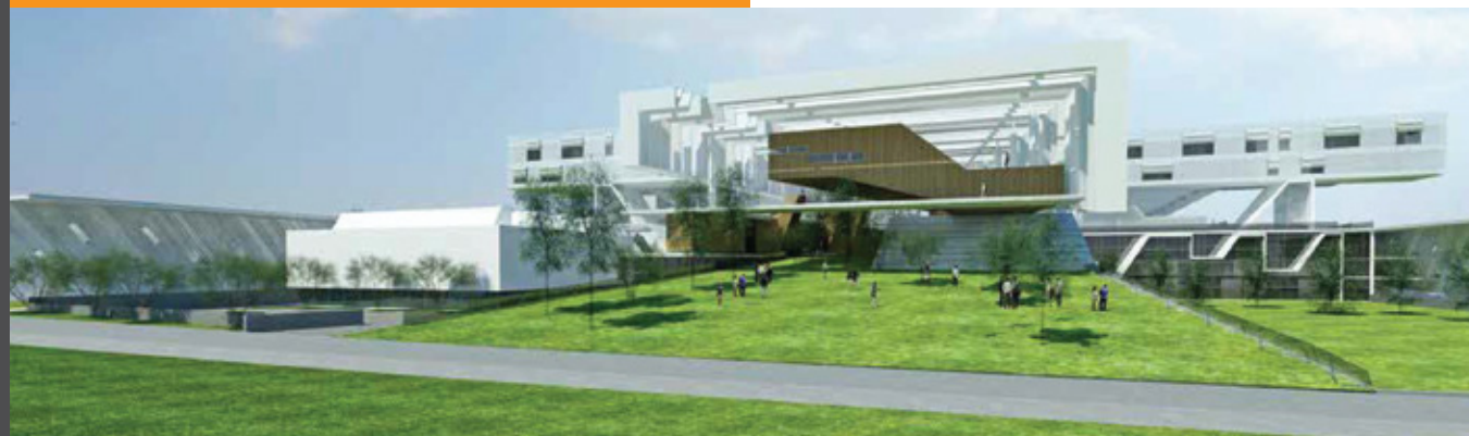
The future building of the UCY School of Engineering which will house the permanent facilities of the KIOS Center of Excellence.
